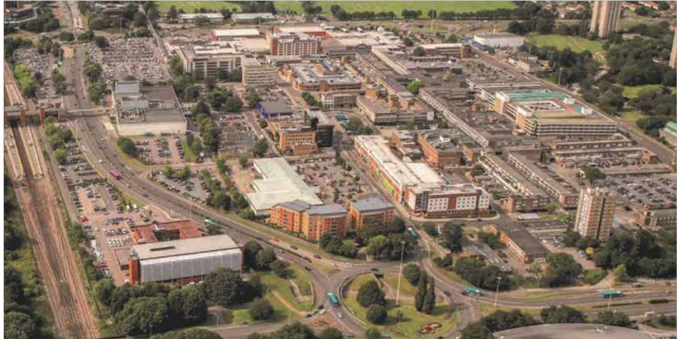
Figure 1: Stevenage town centre from the air
