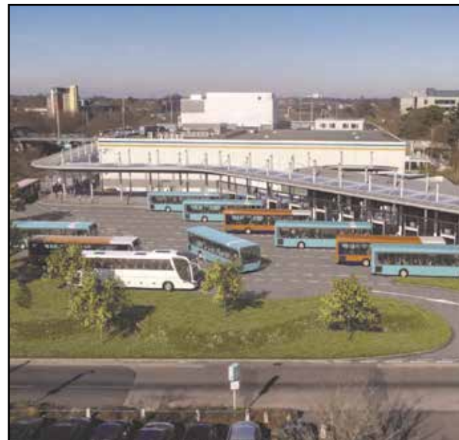
New bus station adjacent to Arts & Leisure Centre
