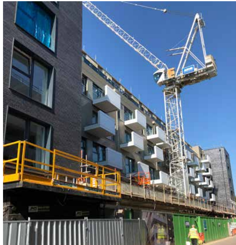
Figure 15: Construction work in Stevenage Town Centre
