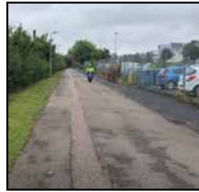
1. Looking north. Police station on right
