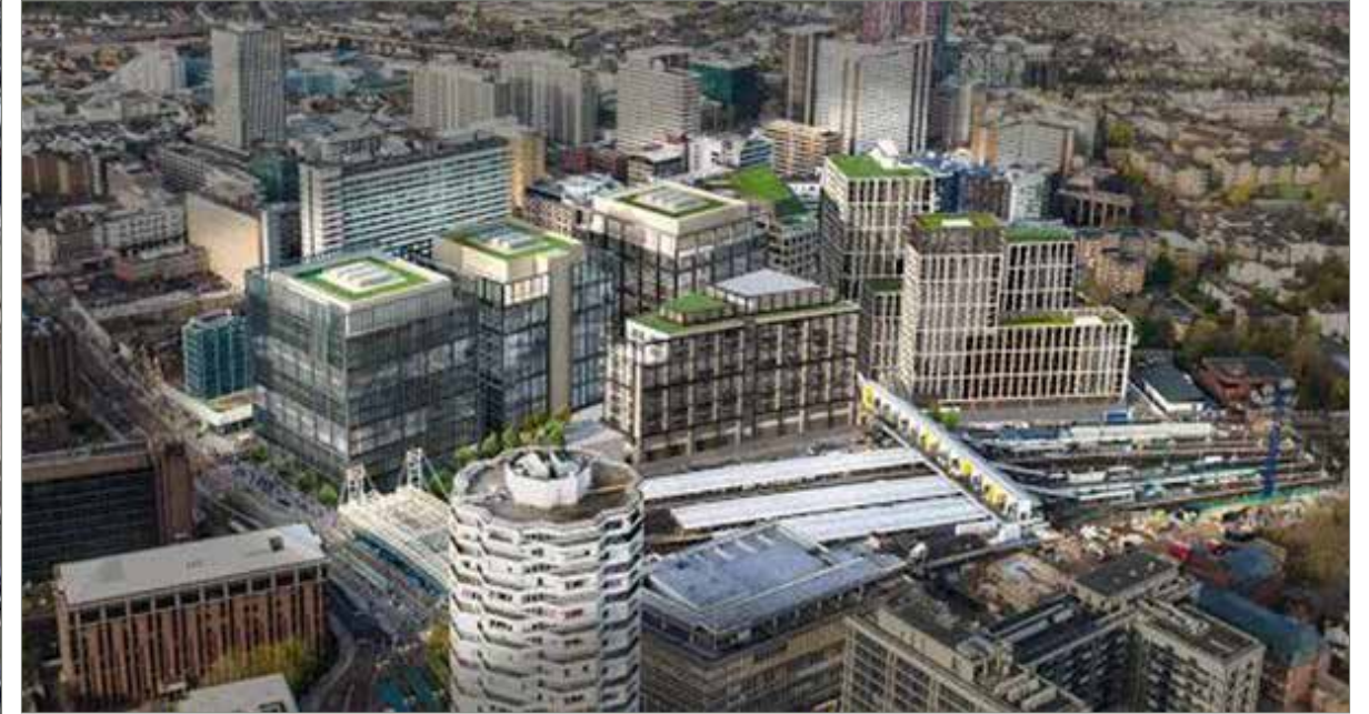
Figure 16: Ruskin Square, East Croydon
