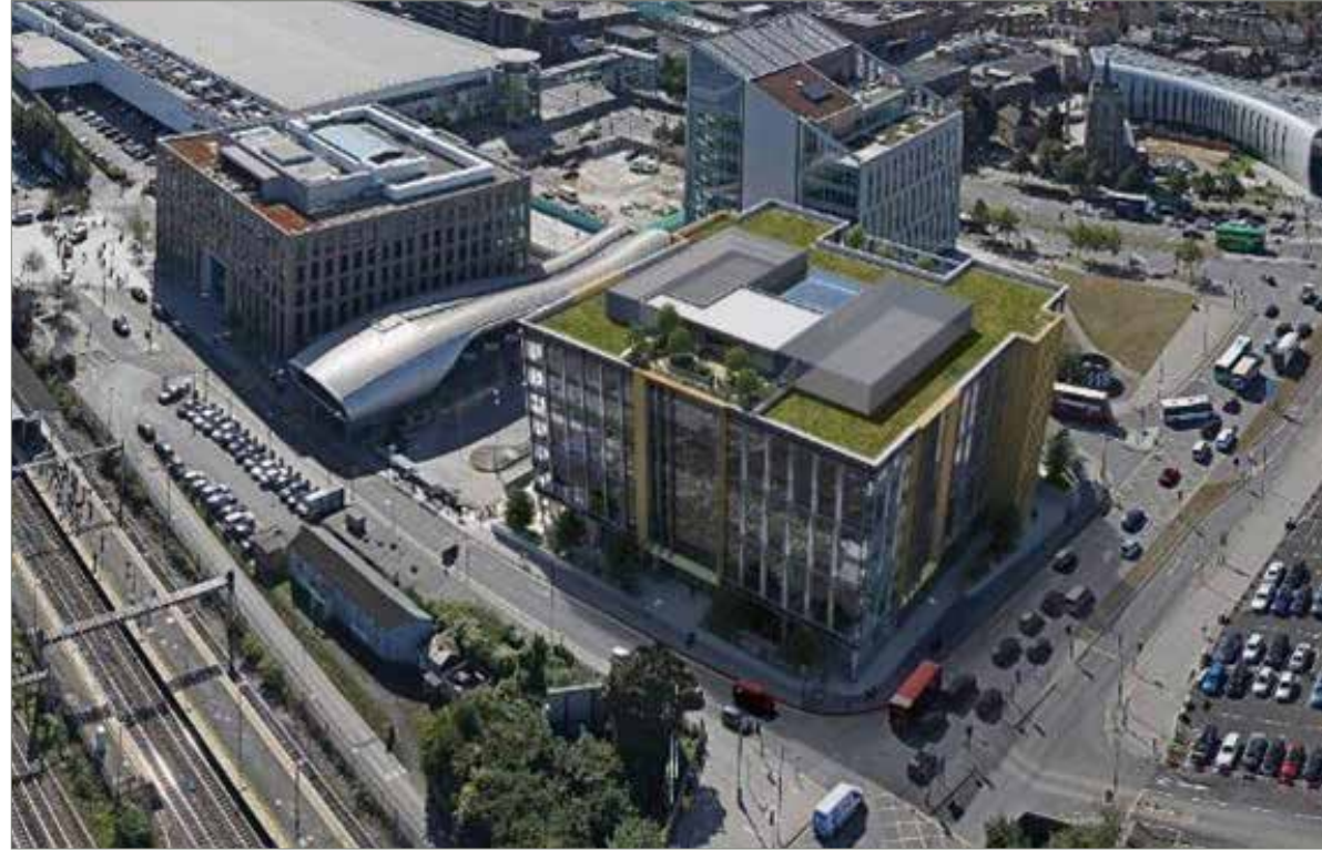
Figure 14: Station Quarter, Slough
